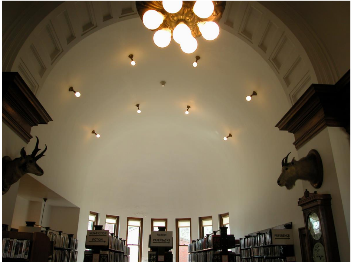
The barrel vault over the stacks.
