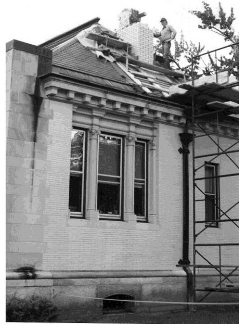
Chimney repair, 1990s.
